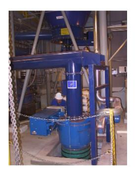
AWS 060530. The bottom of the ash silo, the new screw conveyor and
