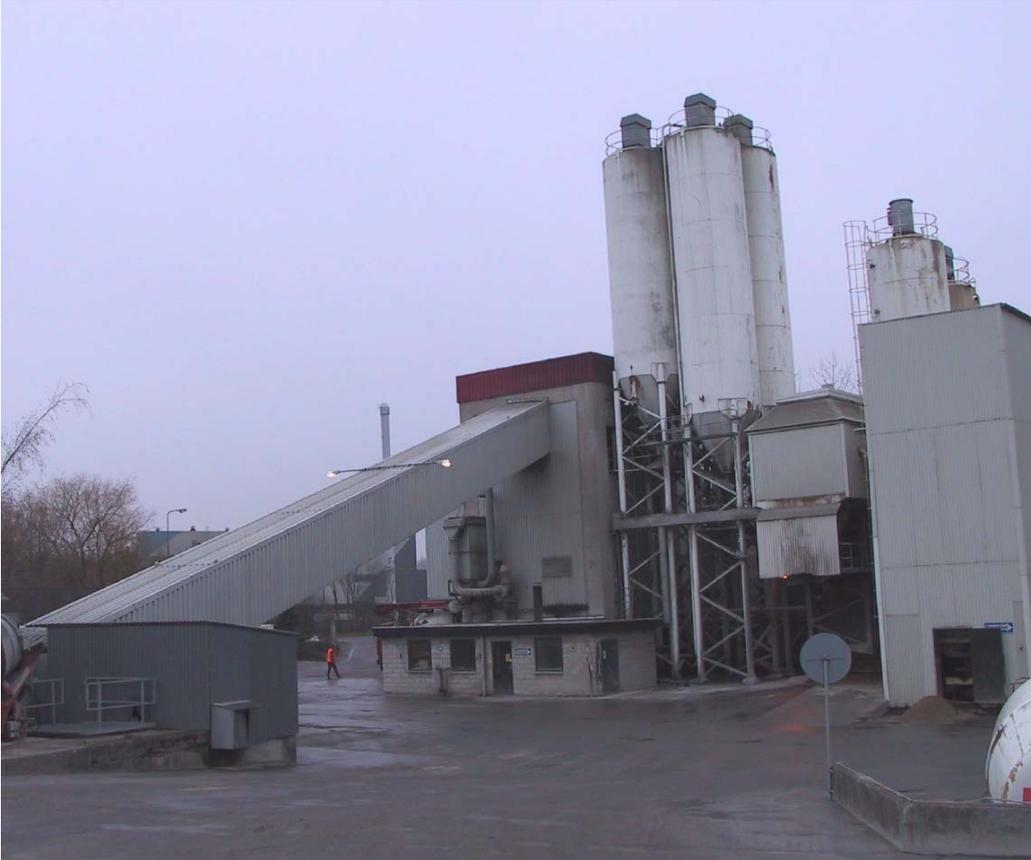
UNICON Ejby 060421. A ready-mixed concrete production plant. One of the high silos has been assigned for the reception of bio ash.
